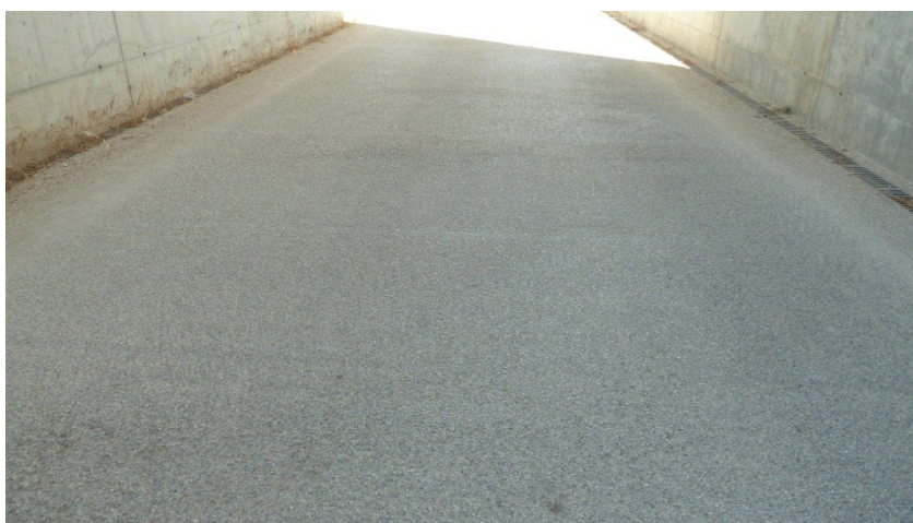
Figure 6. Pervious concrete, roadway pavement
